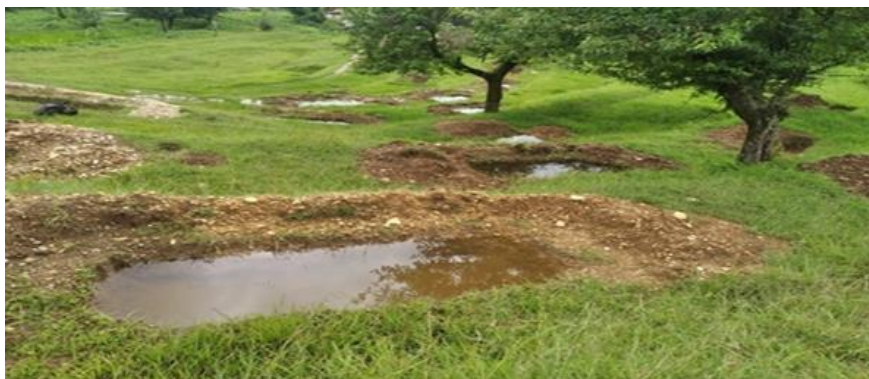
Figure 4: Layout of staggered contour trenches
