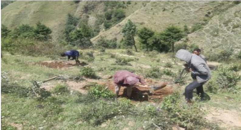
Figure 11: Trenching work in a village
