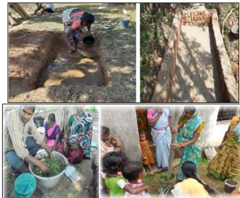
Figure 5.11: Vermibeds construction and vermicomposting
