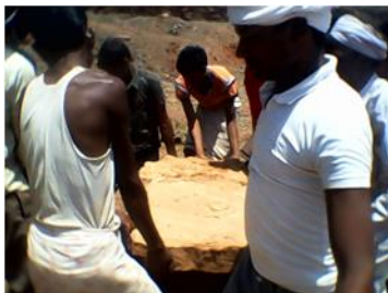
Figure 1.14: Construction of bandstand by shramdan in Bilha tola of Makkepala village
