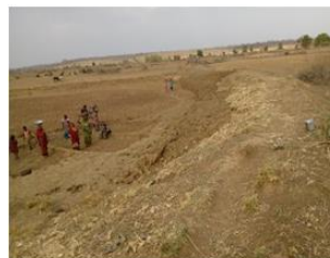
Figure 1.7: Earthen check dam repair
