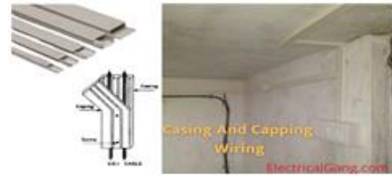
Fig. 10.18: Wooden Casing and Capping Wiring
